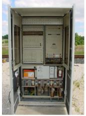
The main feature of signal-protected barrier control equipment is that it gives signals not only towards the public road but also to the railway traffic. It makes a much safer operational principle possible and at the same time it can be operated without supervision.
